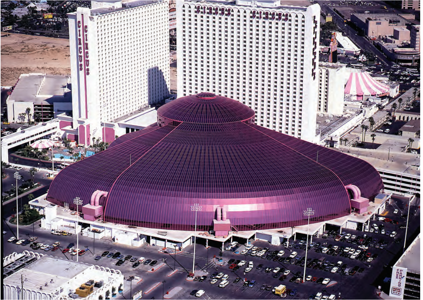
Above: Circus Circus Hotel & Casino, Las Vegas, courtesy of Super Sky Products Enterprises LLC
