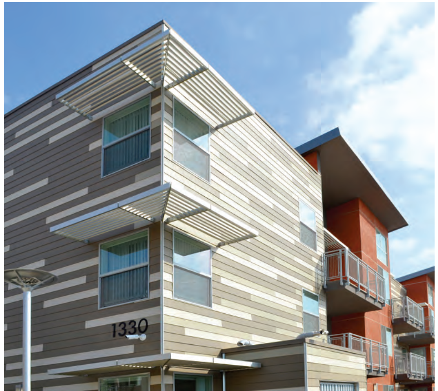
Custom sunshade systems from C.R. Laurence at Sage Park apartment community. Photo by Geoff Captain.
