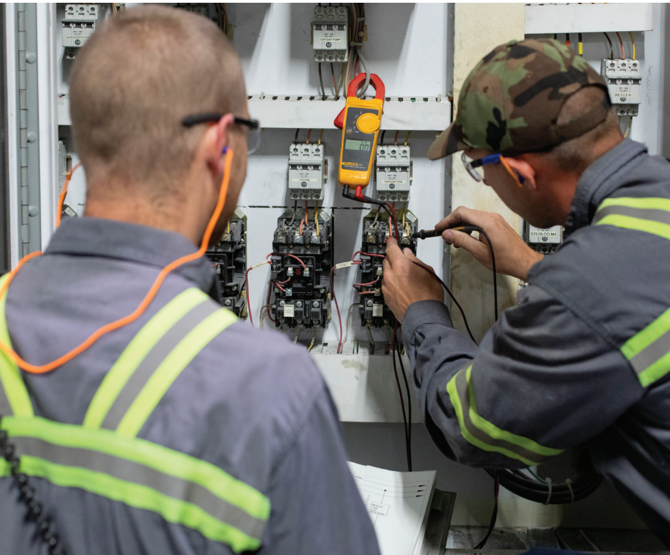
Insulating glass system maintenance at Quanex plant in Cambridge, Ohio. Photo courtesy of Quanex.
