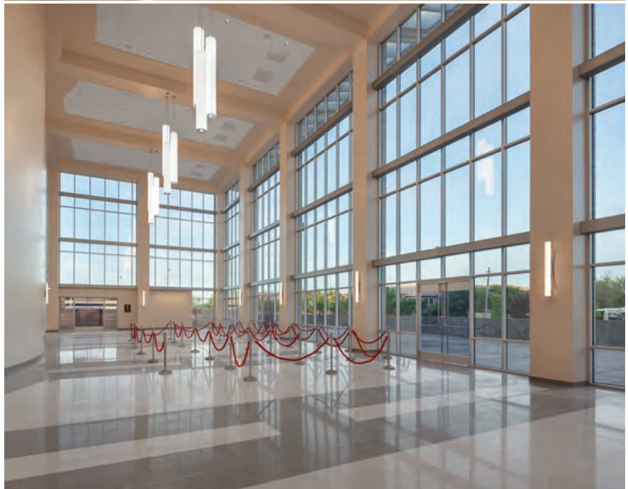
Example of electrochromic glazing in tinted state and clear state. Photos by SageGlass.
