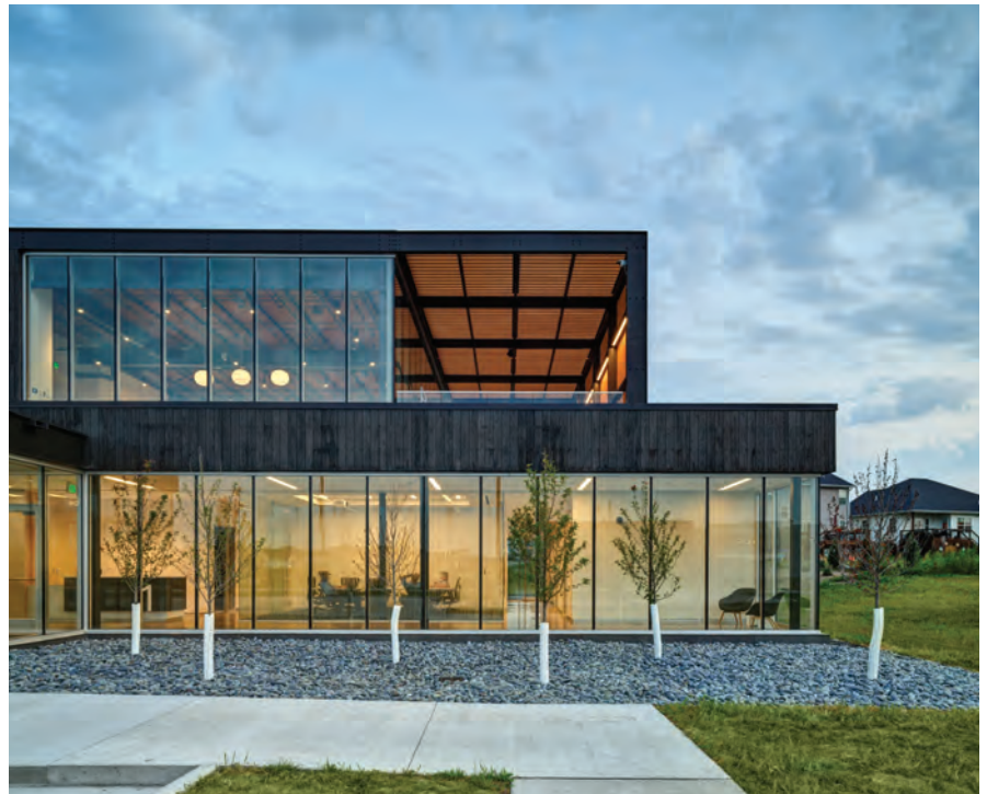
Buildings account for approximately 40% of the total energy use in the U.S. Improving facade performance can reduce building energy consumption. Pictured is the Marion Fire Station in Marion, Iowa, designed by OPN Architects, with low-emissivity glass from Vitro to maximize daylighting and thermal performance. Photo courtesy of Vitro.
